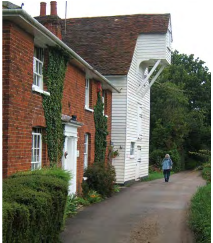
Thorington Mill House and Mill refurbished
